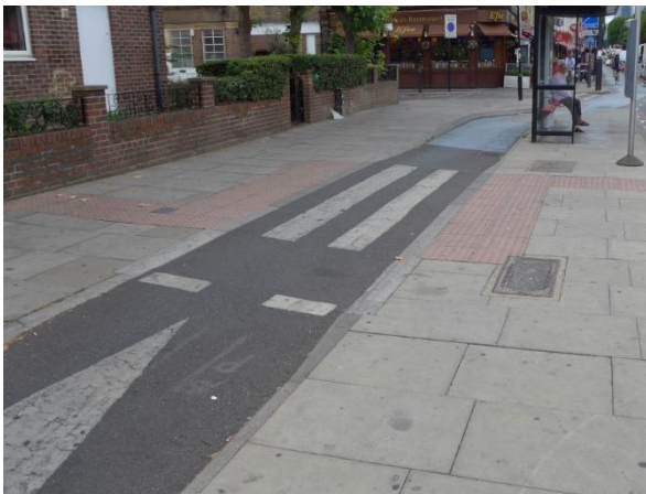
3) Crossing markings lost in a sea of other markings and colour changes
