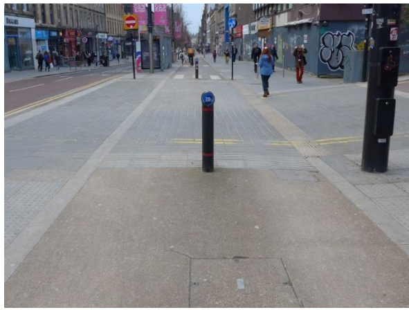
4) Zebra crossings (two close ahead) lost in a complex environment (including a side road crossing)
