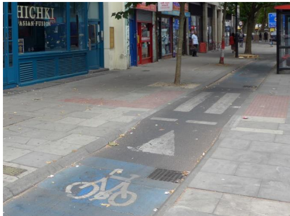
2) Crossing markings lost in a sea of other markings and colour changes
