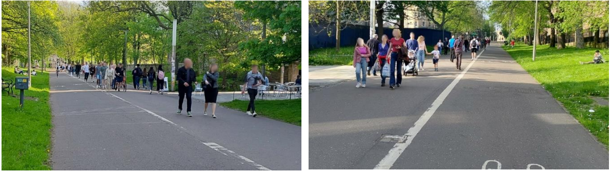
Figure 21: Edinburgh path, separation with painted line
